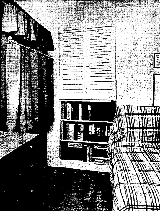
HANDIWORK —Glen built shelves and hung sliding shutters to make unused door into what he calls a "coat and dirty shirt" closet. He mixed paint to match unit to adjacent walls. Chocolate-colored burlap curtains on brass rings were contribution of his mother, Mrs. Steadman Bagby.
